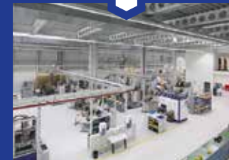
Expansion of production with new 13,000 m 2 production hall
