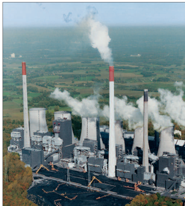
Power plant (EON)
