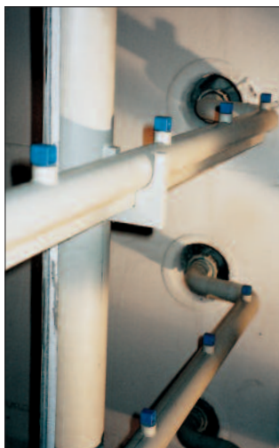
Detail nozzle spray system
