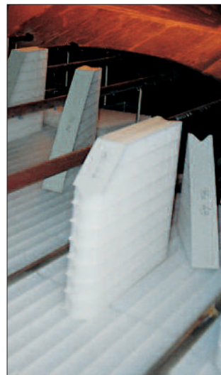
LTV 271 during installation
