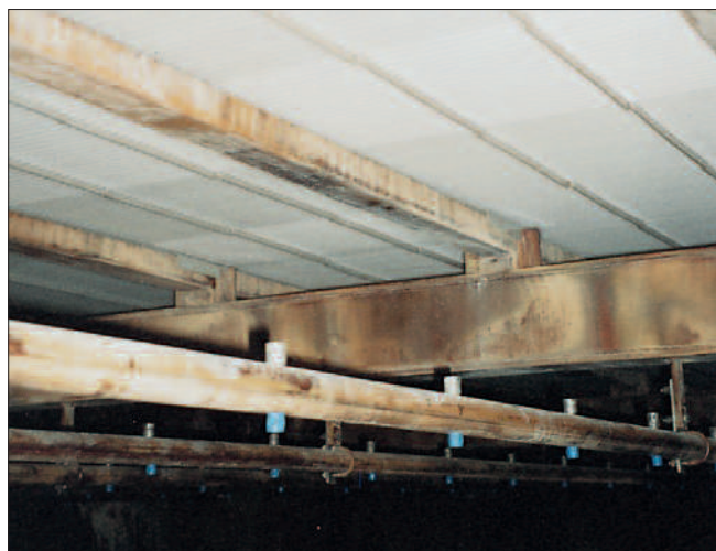
Installed LTV 400 in a flue-gas desulphurization plant
